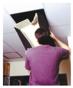
The Luminaire cover has been developed to provide maximum protection for ceilings where fire resistant tiles have been replaced by light fittings.
