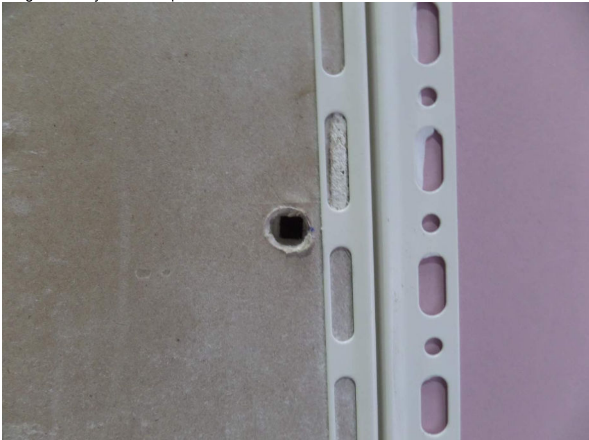
Budget lock key hole on exposed face
