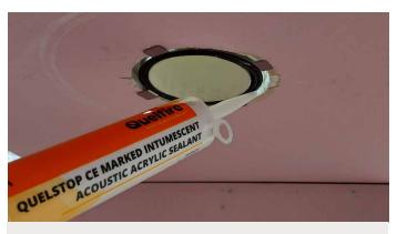
4. Make sure the gap between the CFC100 and the plasterboard is clean of any debris and remove dust from all edges. Seal the small gap between the CFC100 and the plasterboard with QuelStop Acrylic Sealant.
