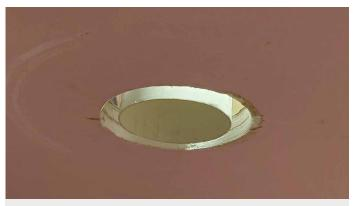
2. Centralise the Ø100mm PVC duct spigot within the hole.
