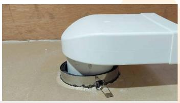
3. From the underside push the Quelfire CFC100 up into the aperture around the PVC duct ensuring the spring clip clamps fully back onto the plasterboard and that the Quelfire CFC100 is clamped tight in position.
