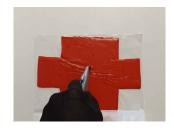
7.a The Putty Pad should completely cover the back and sides of the socket box right up to the front face of the wall.
