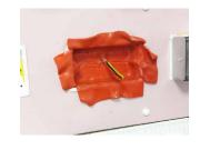
Ensure the Putty Pad is firmly pressed into the whole box and mould the putty back around the cable penetration ensuring that the original 3mm thickness of the putty is maintained at all times.
