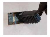
Remove the putty pad from the paper backing and insert the pad into the socket box.
