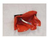
**7.b** Note: where metal boxes are deeper than a standard Putty Pad, additional putty can be added to bring the overall seal to the front edge of the wall ensuring that the original minimum 3mm thickness is maintained at all times.
