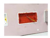
**10.** Confirm the Putty Pad is firmly pressed into the whole box and sealed along the front edge.
