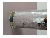
Ensure that the minimum protrusions are achieved check both sides.
