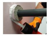
**7.** Where the pipes are required to be insulated, this can now be butted up to the QIF Insulated Fire Sleeve and sealed in accordance with manufacturer's recommendations.
