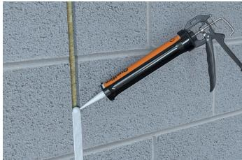
QuelStop CE Marked Intumescent Acrylic Sealant forms part of a lifesaving system designed to prevent the spread of fire through compartment walls and floors, it is therefore essential that the product is installed in a responsible and workmanlike manner with life safety in mind.
