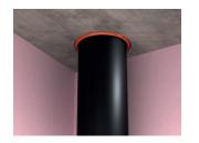
A common misunderstanding is that the wrap protrudes from the underside of the slab but this is **not** a Quelfire tested detail and cannot be rectified if installed in this way. The QWW must be flush with the underside of the slab.
