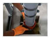
A common misunderstanding is that the wrap protrudes from the underside of the slab/fire protection compound but this is **not** a Quelfire tested detail and cannot be rectified if installed in this way. The QWW must be flush with the underside of the seal.
