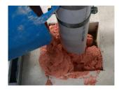
**Q** Use a trowel to ensure the aperture is full and remove any excess QF2 Fire Protection Compound from around the opening.
