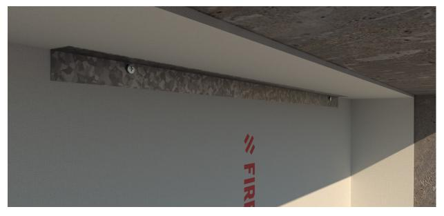
Alternatively the barrier can be clamped in place with a FIREFLY® 25 x 25 x 0.7mm Clamping angle. Fixed with FIREFLY® Panhead Tek Screws as required. This will typically be easier for a two man installation team.
